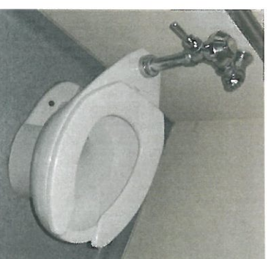
432 flush valve toilets are recommended for replacement with high efficiency units to reduce water usage and limit the impact of anticipated water rate increases.
