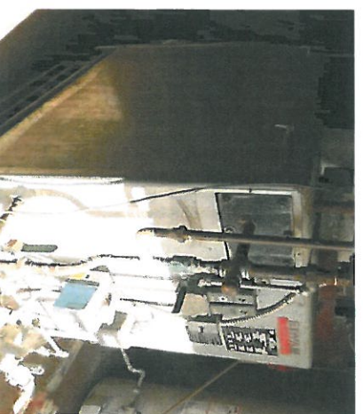
The boiler serving the 2-Pipe system is over 40 years old and oversized for its use.
